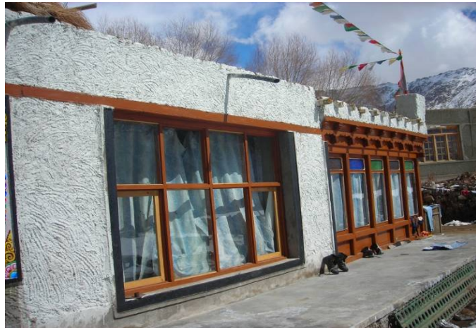
A Trombe Wall for solar passive heating
