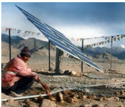
Solar Water Pump
