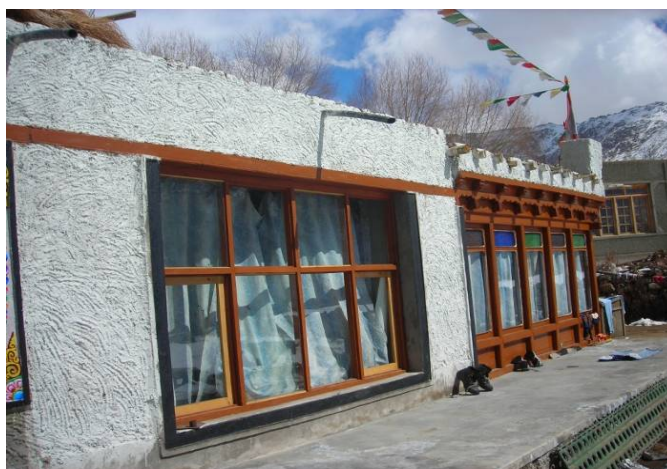
A Trombe Wall for solar passive heating
