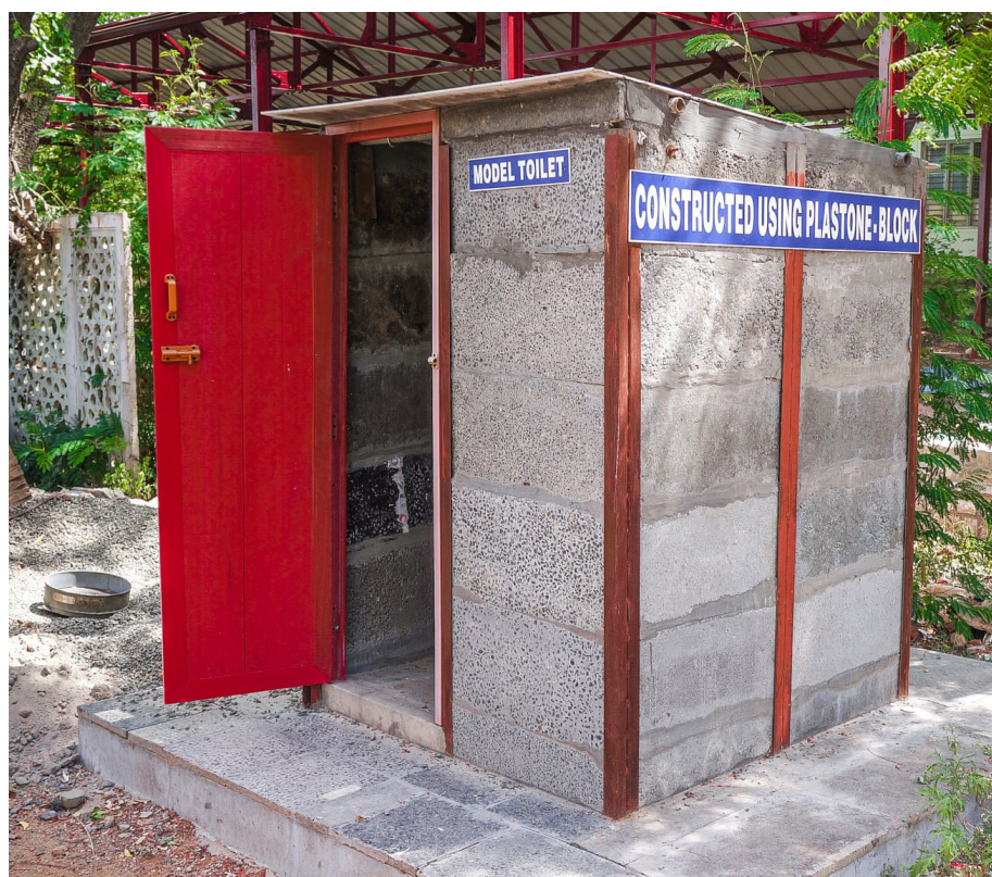
A toilet building built using 'plastone' blocks
